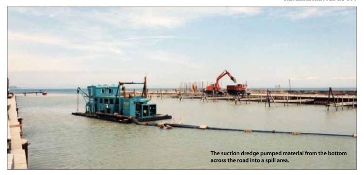
Major dredging of the Point Abino Basin was undertaken in the spring of 1989 in response to record low water predicted for the boating season. Suction dredging was used by Ontario Construction for the job. Soil was first removed by drag line from the berm, trucked across the road and used to create dikes for a dewatering
